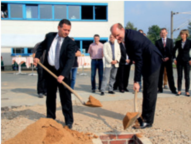
Site manager Steffen Husfeldt (left) and Oerlikon Manmade Fibers COO Georg Stausberg laying the foundation stone for Chemnitz's new R&D center.
